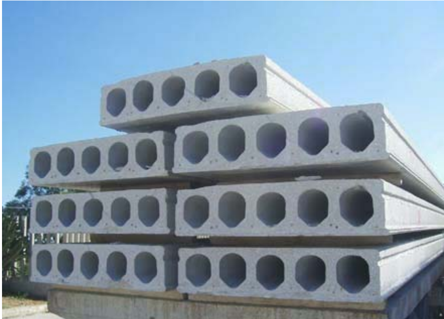
Fig. 7 – Precast Hollow Core Planks
